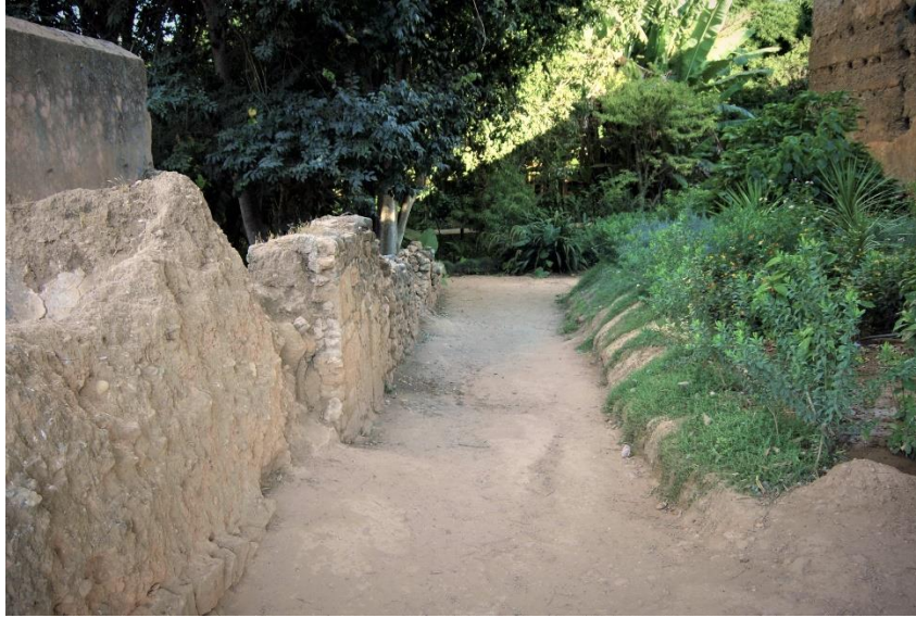
Figure 6. Passage leading to the garden of Shālla, parallel with the north-east wall of the funerary complex. Photo by the author.
