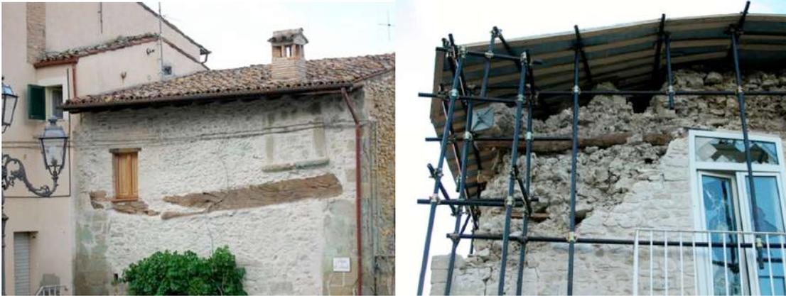
Figuras 3-4. Wooden “reinforcements” (L. Serafini).
