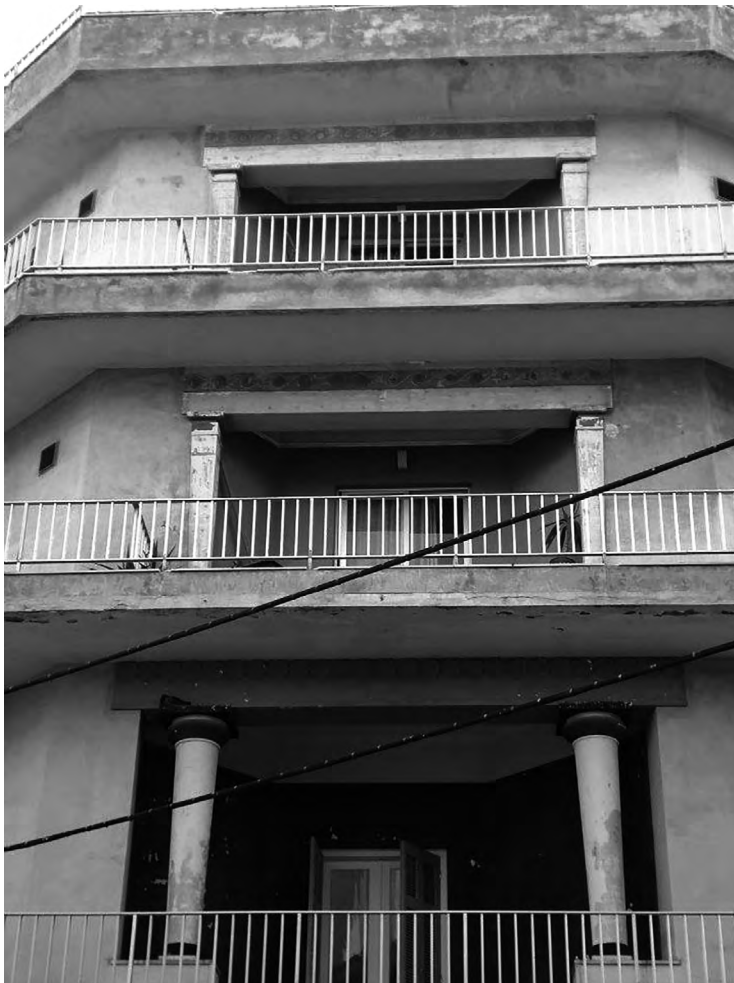
Fig. 3.—Minoan architectural elements in a contemporary building. Heraklion, Greece (Photo credit: Flora Michelaki).
